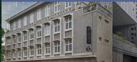
21 Carpenter, Singapore US$74.5m
